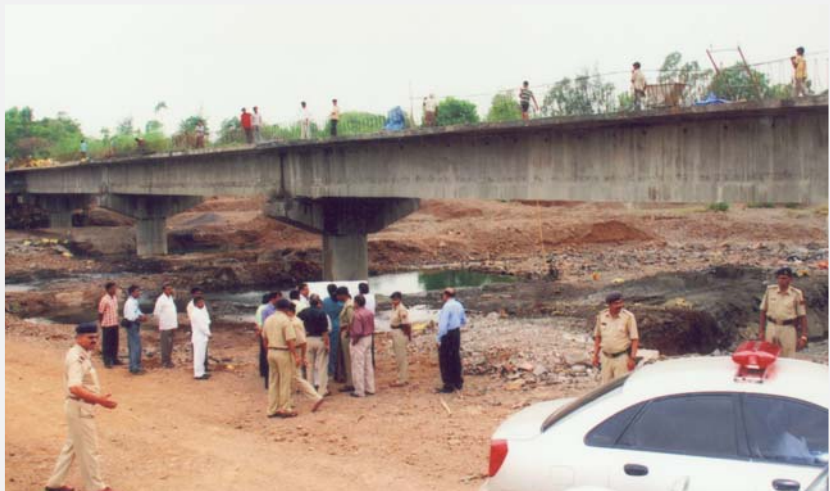
Construction of bridge across rive Sakartod joining Khanvel and Talavali villages, Dadra & Nagar Haveli
