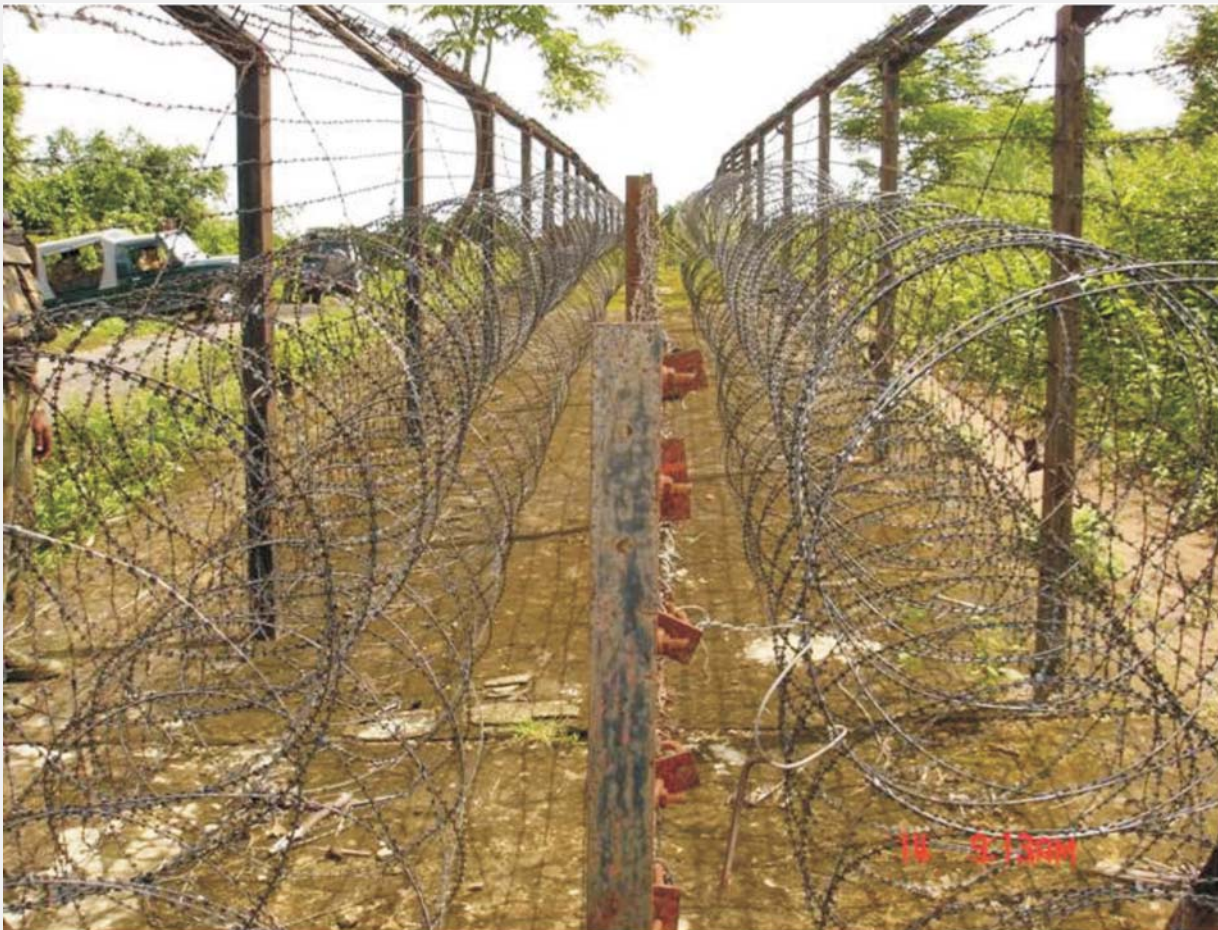
Fencing constructed along Indo-Pakistan border
